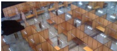
Installation generale de cloisons modulaires
